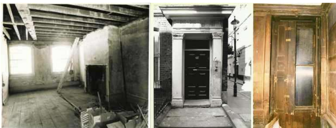
Third floor ceiling removed, front door before stripping 50+ paint layers & ground floor shutters revealed having been nailed in & obscured throughout the house as throughout Meard Street.
