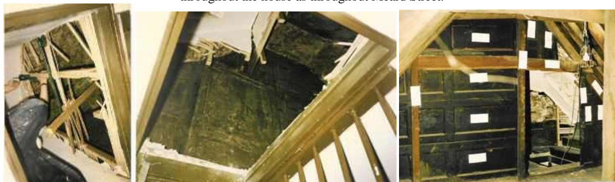
Removing the lathe & plaster to reveal the hidden rooms in the rear attic. Right numbered for removal & restoration.
