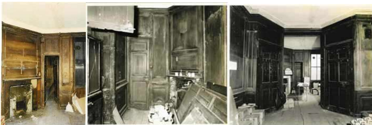
Ground floor before restoration – note missing panelling between the front and middle rooms, now replaced with openable panelling – one panel facing the front room and 4 panels facing the middle room.
