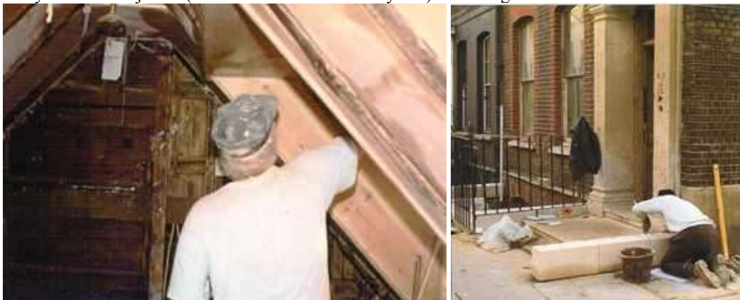
Dave Wise plasterer working on the rear attic 'hidden room'; replacing the missing Portland stone front plinths and door step.
