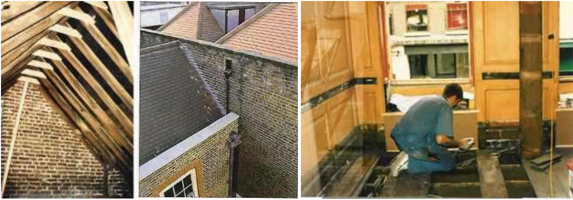
Re-triangulating the attics; rear lead-work flashing; Dean doing electrics after LEB took away the main St. Martin's Electrical Company main board for their museum and ELEC cut my supply. They did not 'Want a dead client before they invoiced me' !
