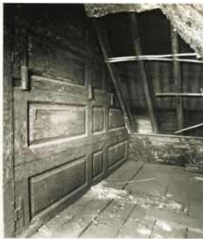
The rear attic 'hidden rooms' – note the 4' high door in the middle pic on the left, skirting and partition both made from window shutters with the latter having a 4' high door still with the original lock.
